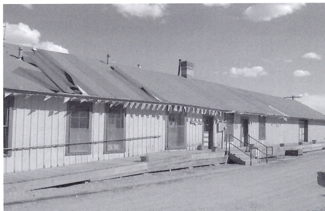
West side of Chama depot roof before repairs, showing deteriorated condition (session A).
