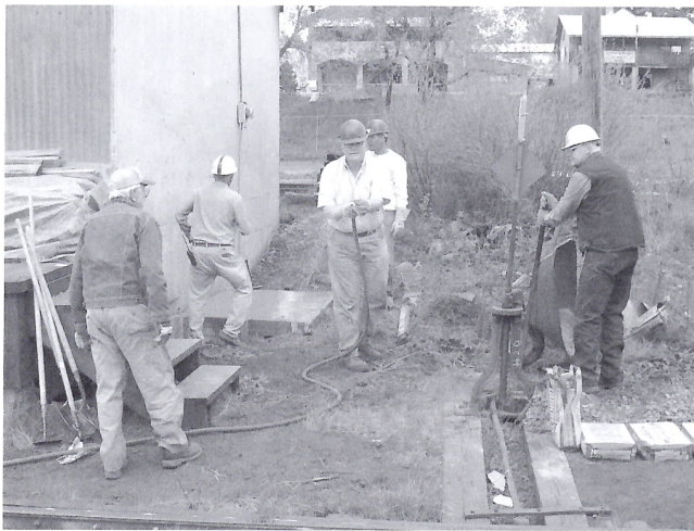
Volunteers have poured the concrete base for the new compressor shed (below) attached to the carpentry shop (session A).
