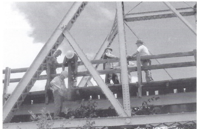
Crew members working on the Chama River bridge walkway and guardrail (session F).
