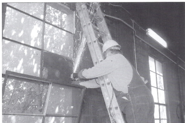
John Manion grinds welded plate from Chama engine house window in session F. Many windows in the engine house were replaced during the August sessions.
