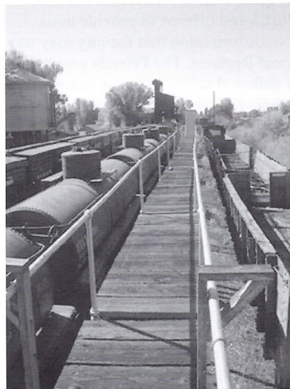
New wood decking and guardrail on the oil storage walkway.
