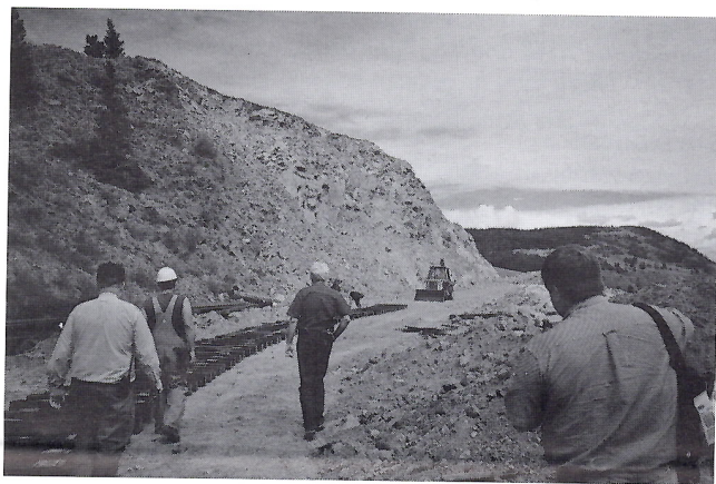
Laying out new ties and track at MP 319, July 2002. The rock blasting area came to the right of the tractor.
