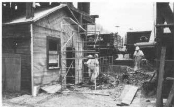
Work began on the coal tippie at Chama. Here, the crew is installing roofing paper on the south wall (the same type of material found on the north wall) of the machinery room after having removed the old and worn-out siding. Some of the old siding was used to repair the north wall.
