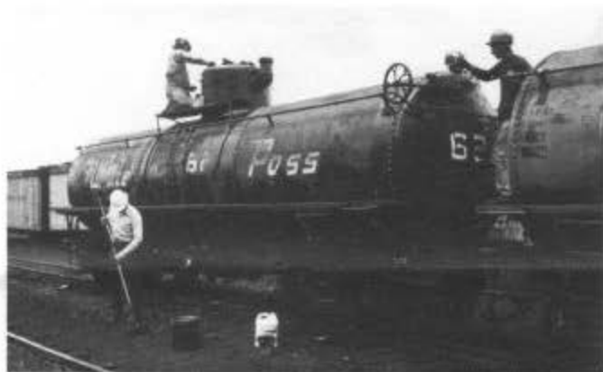
The six tank cars that the Friends purchased from the White Pass & Yukon are parked at the north end of the Chama yard. They were scraped and painted with red steel primer. Here, the crew is working on car no. 62.
