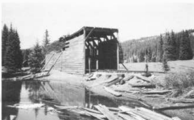
The crew continued the ongoing work of replacing boards and ballens on the sides of the snowshed at Cumbres. Several broken beams in the roof were secured, and three bays were cleared of scrap wood in preparation for roofing at the July/August work session.
