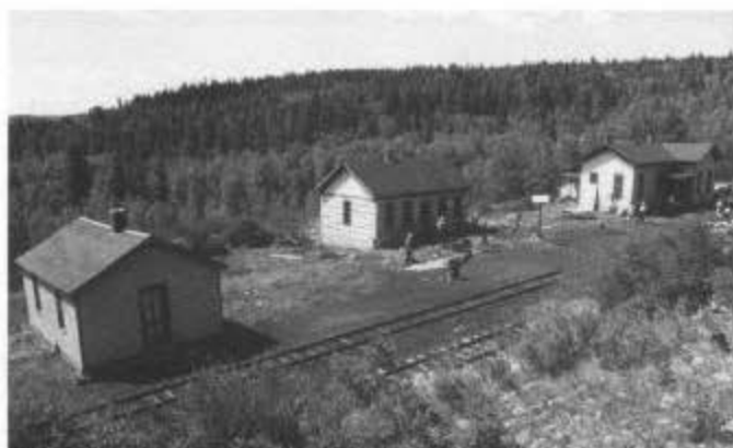
At the end of the work session, the shingle bunk house (left) at Sublette had a new asphalt shingle roof. Volunteers removed the old concrete chinking from the log bunk house (middle). New mortar mix will prevent moisture penetrating into the chinks. The log bunk house also has a new asphalt shingle roof. The section house is shown at right.
