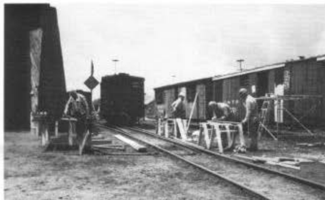
Both interior and exterior work continued from summer 1991 on bunk cars nos. 04258, 04407, and 04982, parked in the Chama yard. In addition to roof and siding work, the crew completed much of the interior work, such as laying and sealing the floors and painting.
