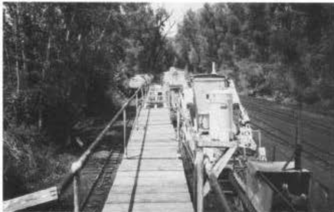
The lower part of the oil dock at Chama was scraped and painted. Aluminum roof coating did a good job in covering the tar that had accumulated over the years on the metal piping. The crew began building a new wooden walkway, and as seen in the photograph, they made a good start.
