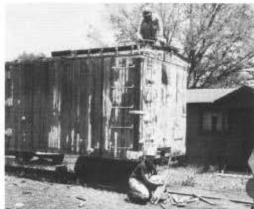
At Chama the 30-foot (short) refrigerator car no. 55 was cleaned, and the car is now ready for repairs. Replacement hardware collected from derelict cars in the east meadow included brake system parts, queen posts, coupler lift bars, and stirrup steps.
