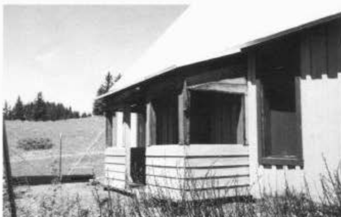
The east porch of the car inspector's house at Cumbres. Volunteers removed the entire porch and then rebuilt it using original materials wherever possible. The porch is now ready for painting.
