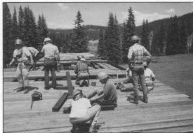
Cumbres: installing new 2 x 12 boards on the snowshed roof over bays nos. 4 and 5.
