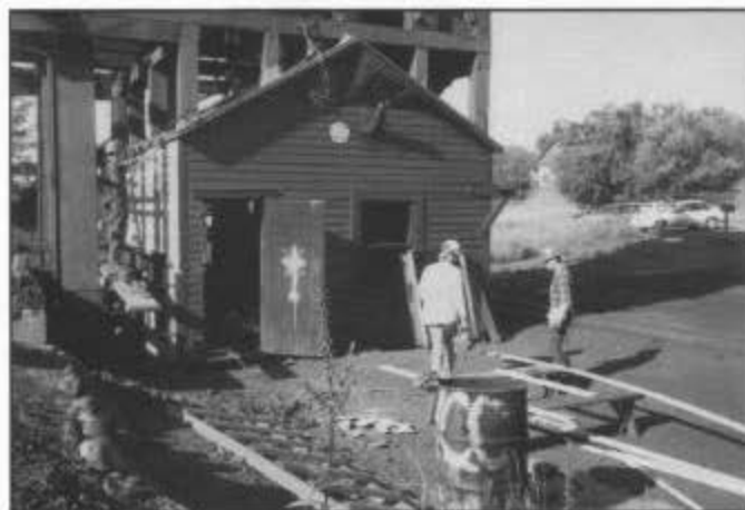
Chama: the coal tippie crew working on the north and east sides of the machinery room; new cedar siding was installed on the east side.
