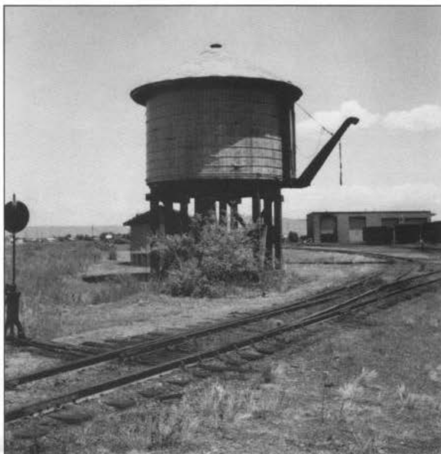
ANTONITO. Looking east, with the engine house in the background. The redwood water tank was constructed in 1977 when the current yard facility was built and is connected to the Antonito town water system. The original (D&RGW) tank in Antonito was located just north of the Rio Grande station in town. August 2, 1992.
