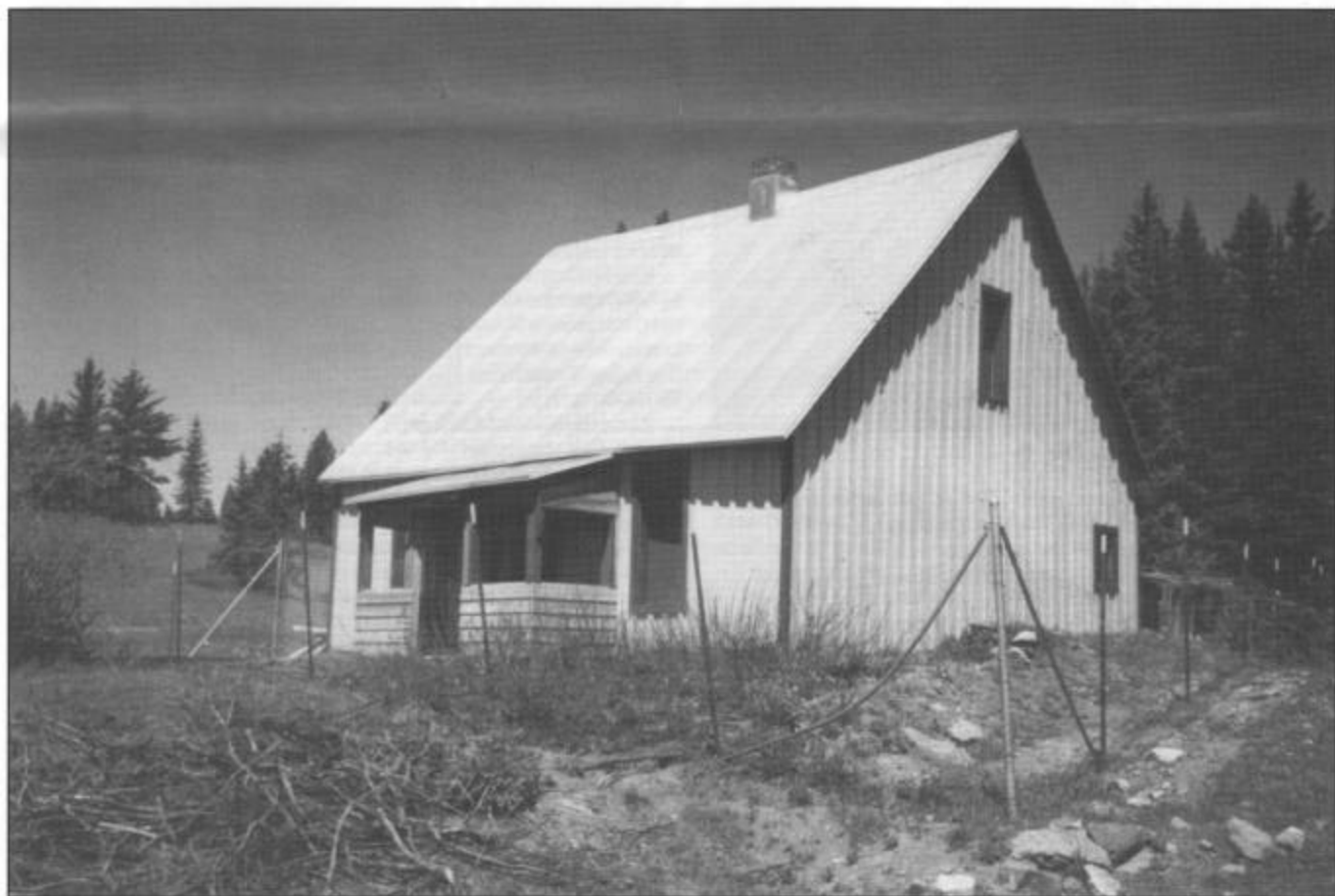
The car inspector's house is shown here in 1992 at the end of the first summer work session. The wooden footing for the front (north) porch had been rebuilt and the porch, with new siding, had been reattached to the house. The final work on the building in 1992 was installing a galvanized metal roof, the cost of which was shared with the Railroad Commission. The building had now been saved.
