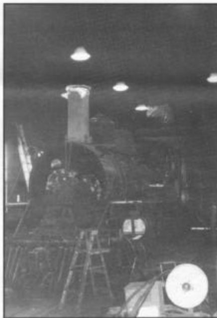
Orlando Ulibarri and Michael Ulibarri work inside 463's smoke box installing the boiler tubes. Note the new sodium vapor ceiling lamps in the engine shop.
