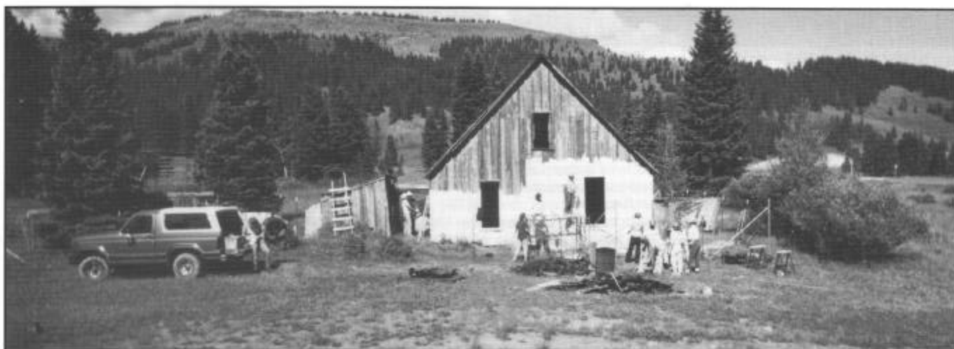
More work was done on the house during the 1991 work sessions. Volunteers completed the south-facing temporary roof and did much work on the exterior siding and battens. They also did many interior structural repairs. The crew is shown here priming the west wall; later they painted the house saffron yellow with brown trim. The snowshed can be seen in the left background.
