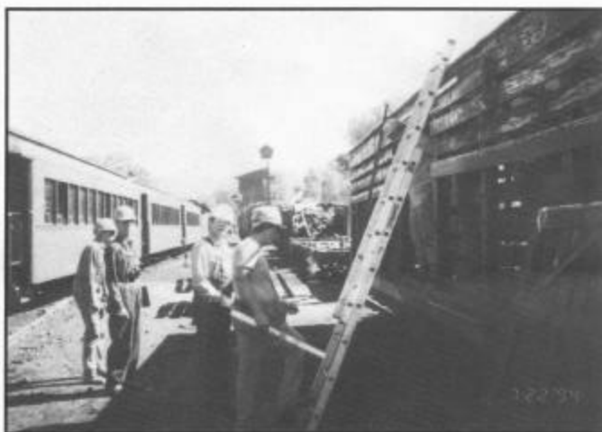
Crew working on the installation of a new roof using historic materials for stock car no. 5691, July 22, 1994.
