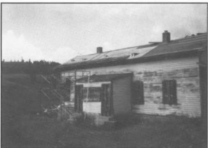
Last year the Osier Section house was stripped of the old layers of shingles and heavy felt paper was put down. This year the beginning of the job saw furring strips placed and wood shingles started, July 20, 1994.
