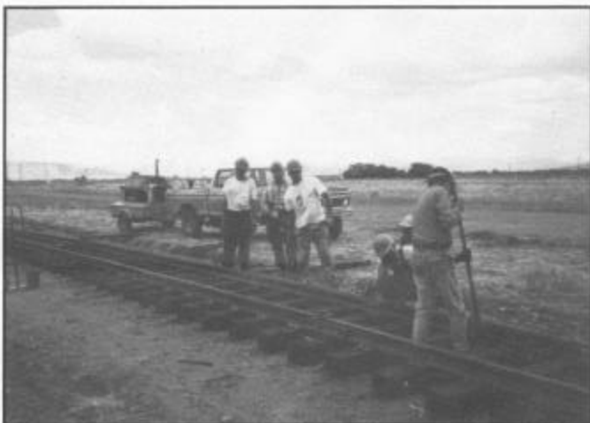
Volunteer crew members look on as final adjustments are made before spiking down the second rail on the new RIP track in Antonito, July 21, 1994.
