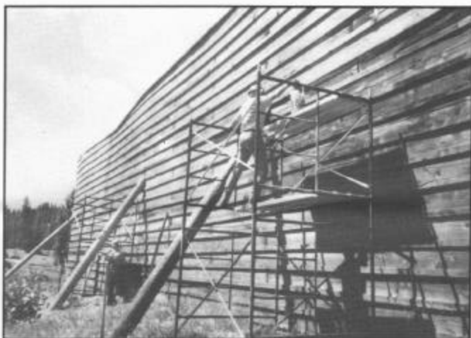
Final touches were put onto the remaining section of the Snowshed at Cumbres Pass. Here volunteers spray linseed oil to help preserve board and batten siding installed over the last five years, July 22, 1994.
