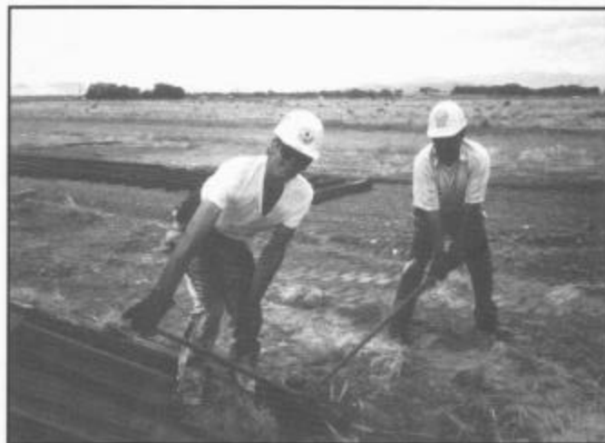
Kyle's track foreman Max Pacheco (right) assists Friends volunteer to lift a rail in preparation for setting it in place on new ties for the Antonito RIP track, July 20, 1994.
