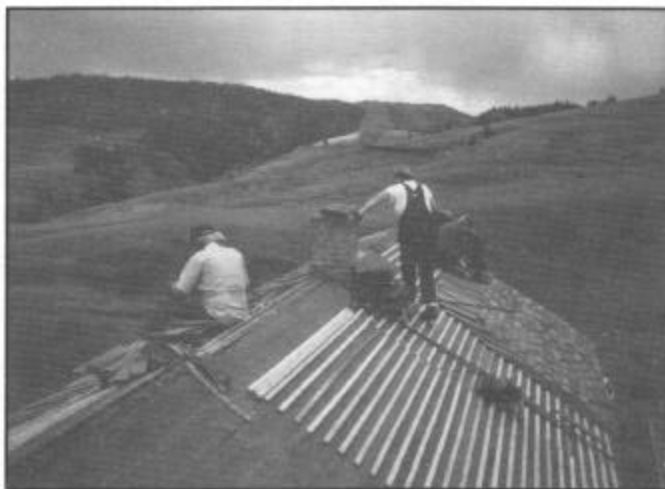
By the last day of the first work session, significant progress had been made on the shingles on the Osier section house roof, July 22 1994.
