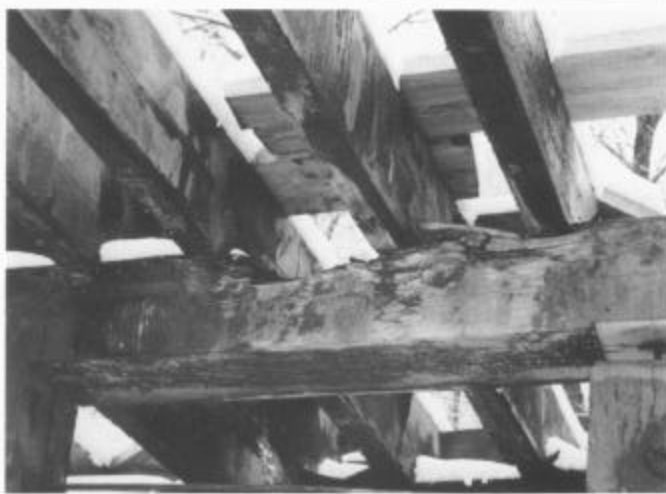
Main beams and chine joists (the wood members holding up the tank floor) showing severe rotting. October 15, 1994.
