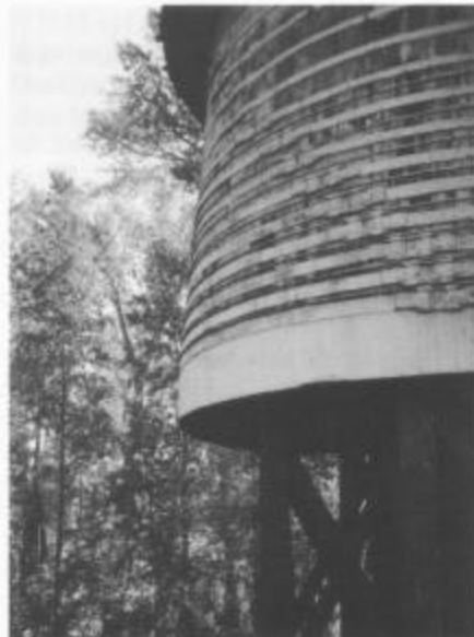
Flat bands with bolted buckles and round bars on the water tank barrel before restoration. September 1993.
