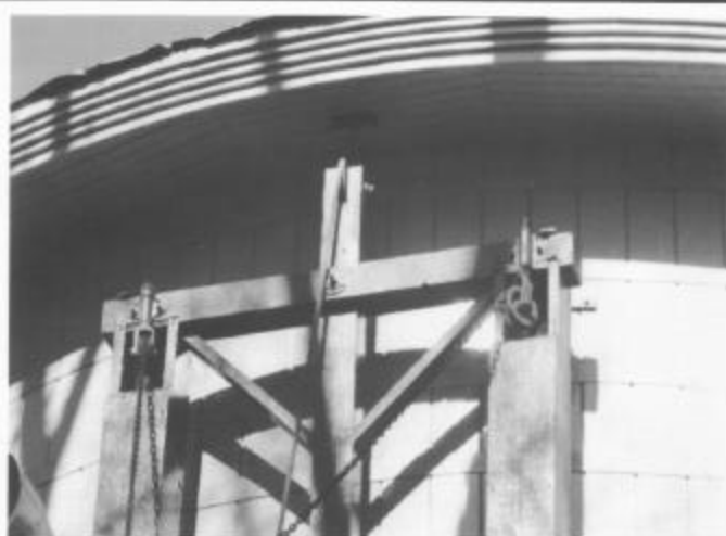
Gallows-type framework for raising and lowering the water spout and opening and closing the interior valve. June 1995.
