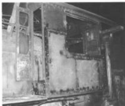
Inside the engine house major work has been going on with 488 throughout the winter. This view from January 22, 1996, shows the new sheet metal siding on the engine's cab.
