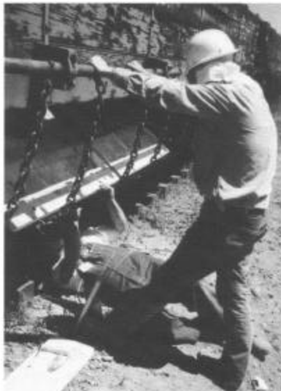
Repairing doors on a drop-bottom gondola during the 1995 summer work session. August 1, 1995, Antonito, Colorado. Photo by George Swain.
