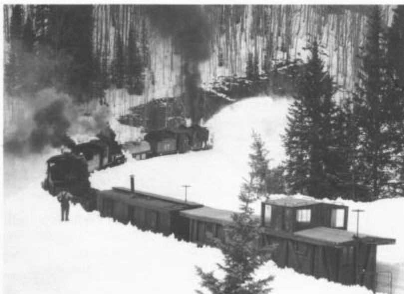
Rotary OY between Coxo and Windy Point on May 10, 1995. The snowplow was pushed by engines 487 and 489. Photo by N. G. Wilson.
