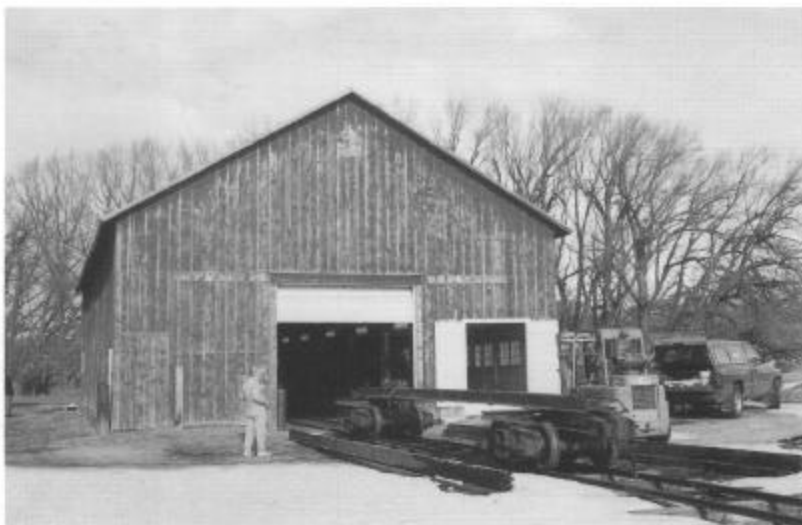
In order to have an enclosed work space, volunteers put down track in front of and inside a nineteenth century dairy barn on museum property, and museum staff installed new light fixtures and electrical outlets. On January 3, 1998, flat car 6200, stripped of all wood and showing the steel center sill, body bolsters, trucks, and couplers, was parked on the track. Art Nichols photo.
