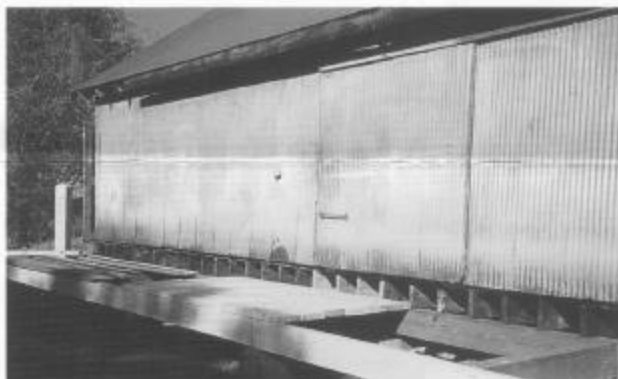
New sill and platform supports for the Chama warehouse loading dock (session B). George Swain photo.
