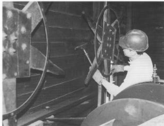
Clyde Putman vacuums the wall of the hoist house. Coal dust has to be removed before paint will adhere to the walls (session A).
