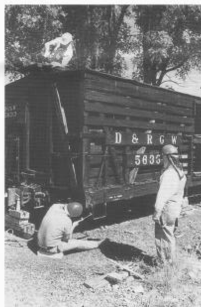
Replacing the end sill on stock car 5633 in the Chama yard. Geof Gordon on the roof, Steve Broadhurst with the torch, and Gary Rauch (session B).
