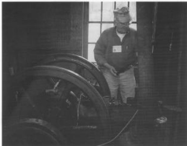
The Friends plan to restore the Chama coal tipple, built in 1924, to historic and operating condition. Restoration began this summer with a general cleaning and inspection of the hoist house. During session A, Parker Fowler inspects the one-cylinder Fairbanks-Morse engine with cable drum, not used after an electric motor (GE, 10 hp) was installed. George Swain photo.
