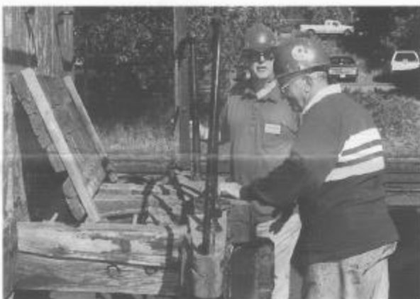
Donald Storm and Dave Sands survey the condition of the wood in the end platform of cook car 053, Chama, June 1997. Tom Cardin photo.
