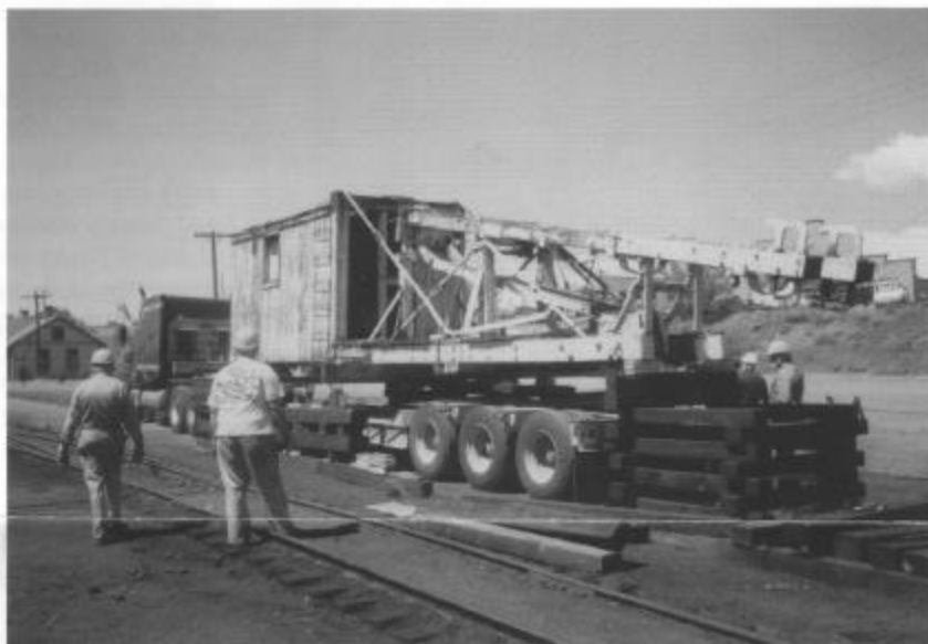
Pile driver OB's superstructure is lowered onto a flat-bed truck in the Chama yard on June 24, 1999. OB's flat car upon which the superstructure rests has been removed. The pile driver, built in 1891, was taken to the Friends' facility at the Western Museum of Mining and Industry at Colorado Springs for restoration. (George Swain)
