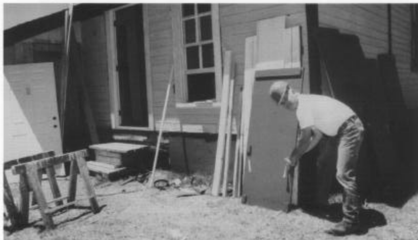
Volunteers completed the new porch roof of the Osier section house (session B). Below, Rich Muth works on window covers for the Cumbres section house. Note the new door and new window frames and sills (session B).
