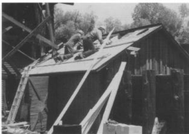
Reroofing the sand house, next to the coal tippie. Fire damaged part of the earlier roof, which the Friends installed in 1997.
