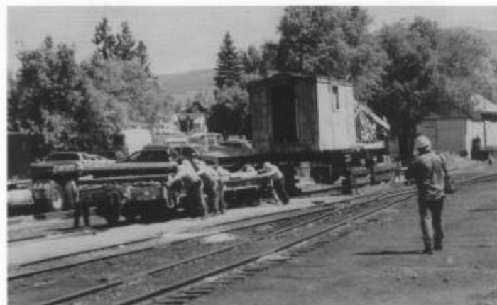
After OB's superstructure (pile driver frame, tower, hoist machinery and hoist house) was raised with jacks and supported by cribbing, the flat car was rolled out from under the superstructure (session B).
