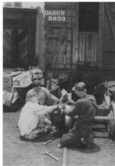
In Chama, Charlie Irvin (sitting), Jack Salisbury and Don Hausmann work on a bearing box from stock car 5633 (session A).
