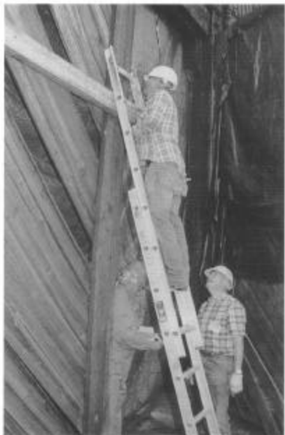
Bob Tully positions a plank on the Chama roundhouse door so it can be lifted off for repair. Terry Boardman (left) and Roger Briggs survey the situation (session D).
