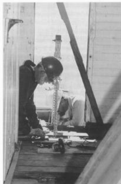
Warren Ringer (left) and Tom Garland work on short caboose 0579 during session D. They use an hydraulic lift to bring the bolster up and hold it while it is bolted in place.
