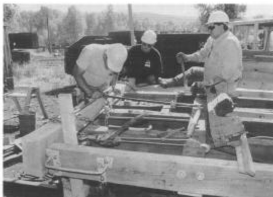
In the Chama yard during session C, Roy Blizzard (left) and Dave Sands guide the end sill on to wheel and tie car 06092 while Tony Kassin uses a come-along to draw it into position.
