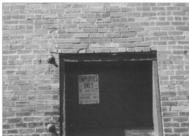
South doorway of Chama boiler room and machine shop. The single brick of the original arched doorway is above and to the left of the door. (Photos by Tom Cardin)
