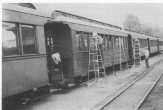
Putting final touches on coaches in preparation for opening day. Three coaches in Chama were painted. On the exterior of all the Chama coaches, loose panels were repaired and all the trim was tightened.
