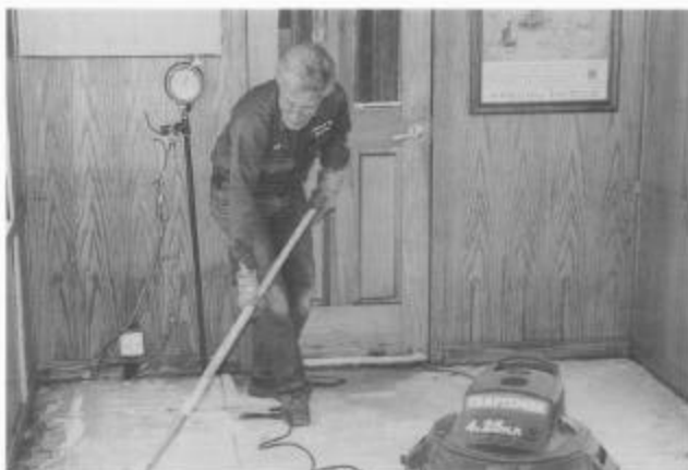
Bob Ground removes the old linoleum from Chama coach Cumbres. Volunteers then installed a new floor. They also replaced broken windows and repaired seat mounts.
