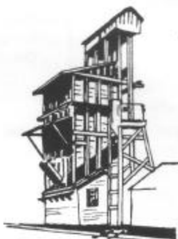
12. Coal Tipple. It was built in 1924 to replace an earlier inclined coal trestle. Cars carrying coal would be pushed onto the Coal Loading track on the east side of the tower. The coal was then dumped into bins. Coal was then hoisted from . . .
