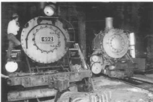
During session B in June, engines 492 and 483 await asbestos removal in the old roundhouse in Chama. Clyde Putman is on the running board surveying the piping and other attached parts. These parts were removed in session D. (Tom Cardin)
