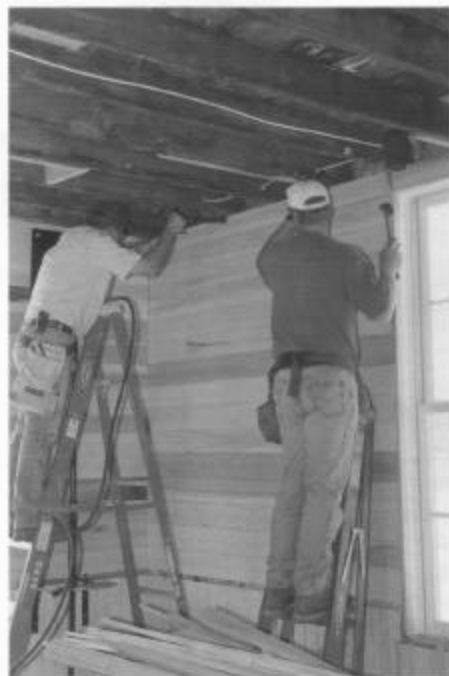
Inside the Osier depot, Dan Robbins (l) and John Ruhr fit the final beadboard strip on the wall of the first floor. The chair rail and beadboard on the ceiling are yet to be completed (session B). (Photo by Sheri Hamblin.)
