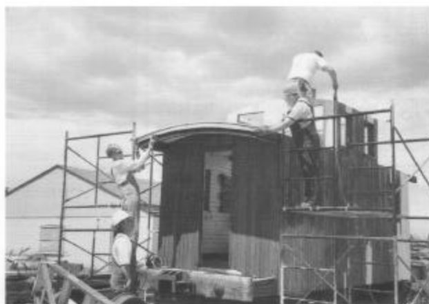
In Antonito during session A, Warren Ringer (l) and Jim Rhinehart install a curved "nailer" board on the roof end of short caboose 0579. Bill Kepner on the ground helps center the board, and Charlie Irvin works on the cupola. (Photo by Art Nichols.)
