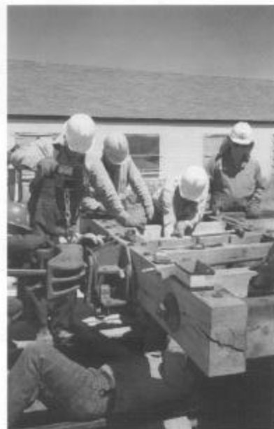
In the Chama yard, Tim Bristow (l) and George Detwiler replace the interior siding of boxcar 3605 during work session B. At right, in Antonito during session B, from the left, Warren Ringer, Jim Laycock, Jack Salisbury, Norman Grant, and Keith Hayes install a coupler on idler flat car 6708. Art Randall works under the car. (Photo by Art Nichols.)
