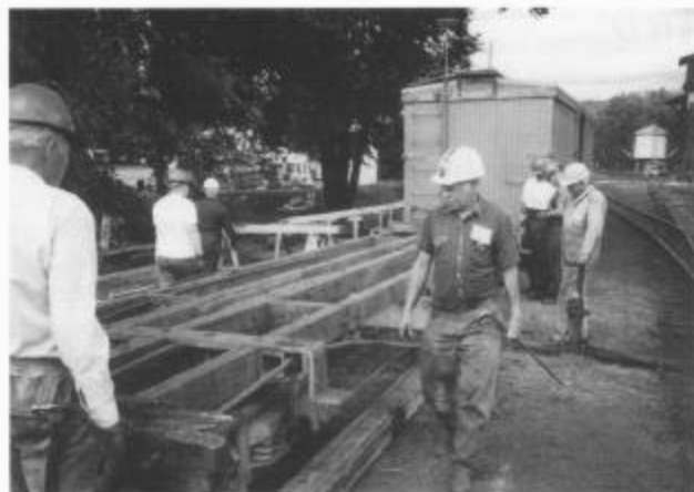
On the final day of session C at Chama, Bob Tully inspects boxcar 3339 (former coach 200) with side sills removed. (Photo by George Swain.)
