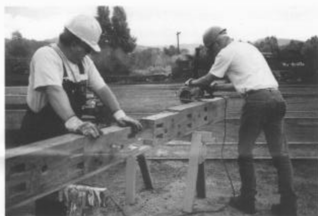
John Manion (l) and Richard McLean prepare an oak end sill for boxcar 3339 in the Chama yard, session D. (Photo by Terri Shaw.) Below, Walt Sommer (l) and Dick Seelye work on the table saw while Ron Schmitt uses the miter box and saw in the Cumbres section house during session C. (Photo by Tom Cardin.)
