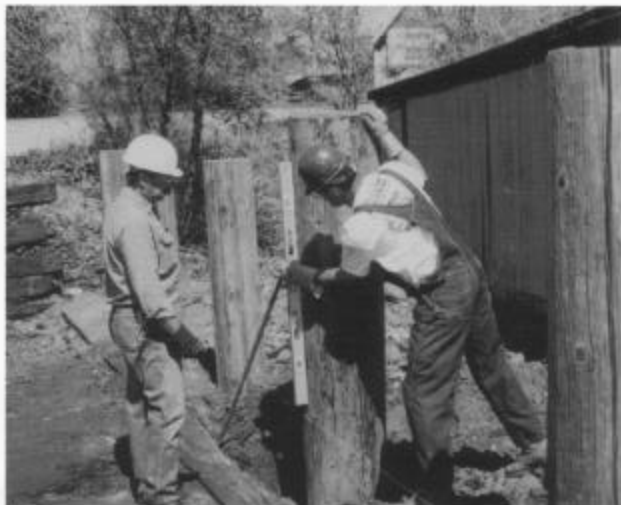
Jerry Sahnd eyeballs, while John Sutkus uses a level to set posts for the coal bunker in the Chama yard (session B). Emery Maez, general manager of Northern Rio Arriba Electric Cooperative, provided a truck and crew that drilled the holes for the posts, 16-inch-diameter, used, telephone poles that had been in the north yard. (Photo by Tom Cardin.)
