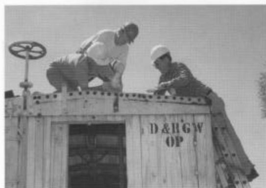
Dick Seelye (l), Grant Harrison, and Charles Joerg remove plumbing from the top of derrick OP so that they can put down weatherproof roofing material (session F).
