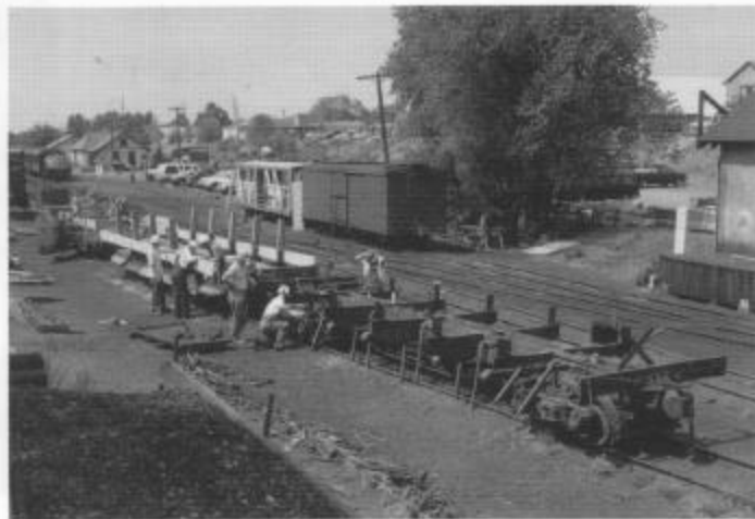
Drop bottom gondola restoration underway in Chama during session C. To the left is car 791; the crew starts to install new doors and siding. To the right is car 811 stripped to the metal frame. Boxcars 3339 and 3605 are in the center background.
