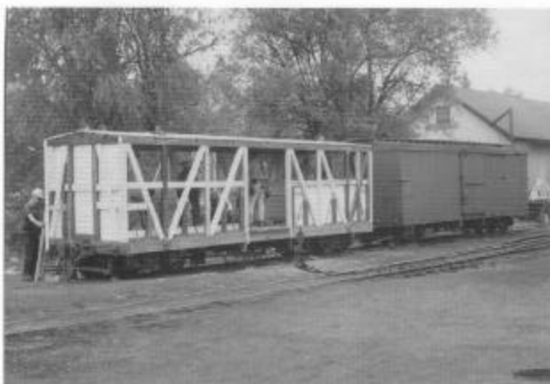
The conversion of passenger coach 200 back to its original 3339 boxcar configuration underway in the Chama yard during session C. Next to 3339 is boxcar 3605, converted from coach 209 in 2001 and ready for lettering.
