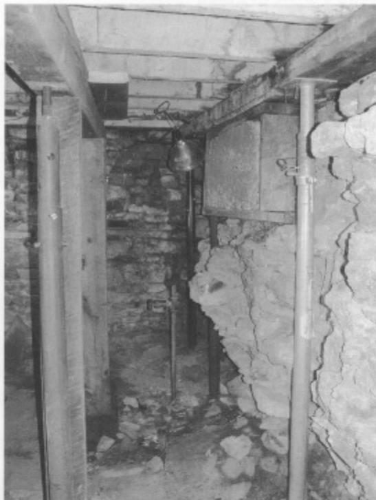
*This photograph shows three of the four jacks supporting the base sill (right) and one of the jacks and cribbing supporting the floor joists (left). The dark colored jack in the back (east end of base sill) was installed this summer during Session C. (Jim Herron)*
