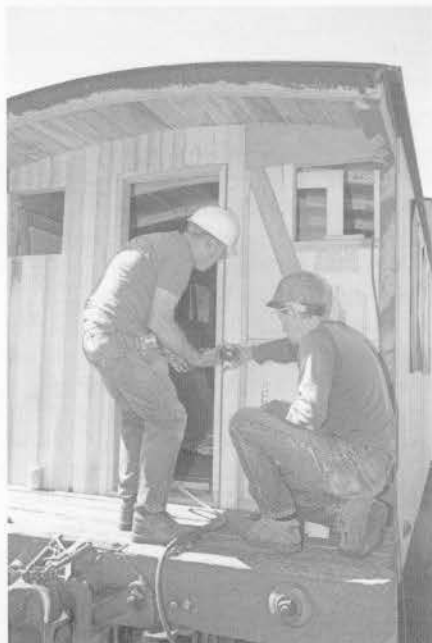
Ron Schmitt and Norval Alliston put siding on caboose 05635. (Tom Cardin)
