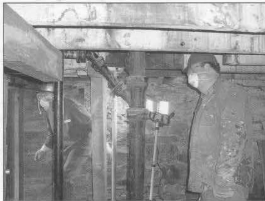
Dick Seelye and Team Leader Jim Herron working to get jack post ready to install. (Chronicler photo)
