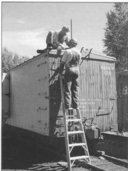
Matt Jameson and Pete Hogan (on ladder) installing a retainer valve and pipe. (Chronicler photo)
