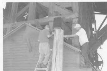
Samuel Schechter and Wendel Scwietzer place a plastic membrane on the coal tittle to protect from falling ice. (Tom Cardin)
