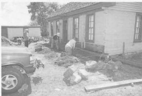
Using the winch to move the 12x12 30-foot-long beam under the log bunkhouse. (Tom Cardin)
