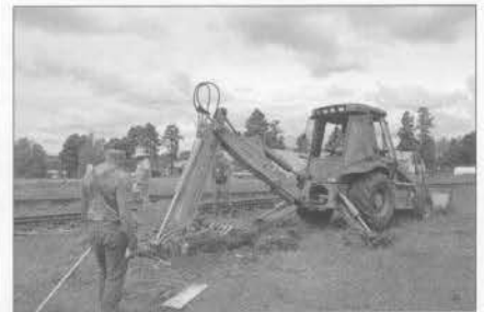
C&TSRR Chama Shop Foreman Steve Montano, in backhoe cab, digging one of the eleven holes for installation of the telegraphphone poles. Left to right, Ron Horejsi, John Cole, and Skip Hillegas observe. (Chronicler photo)
