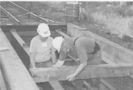
Daryl Locker and Frank Smucker install a tie on the scale. (Tom Cardin)
