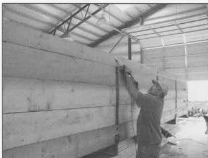
Bob Osborn uses a sawsall to cut a bolt off even with the nut.
