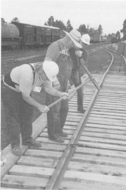
Daryl Locker and Bob Anderson watch as Frank Smucker spikes down a rail on the scale track. (Tom Cardin)
