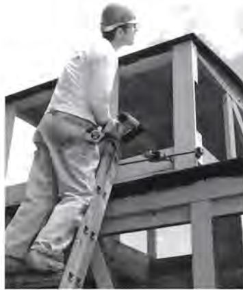
John Sutkus fits the first piece of sheathing on the cupola.
