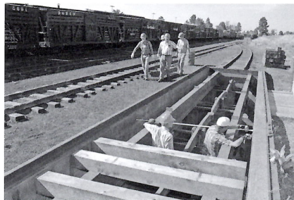
The miscellaneous repairs team sets ties on the scale in preparation for temporarily covering the pit.
