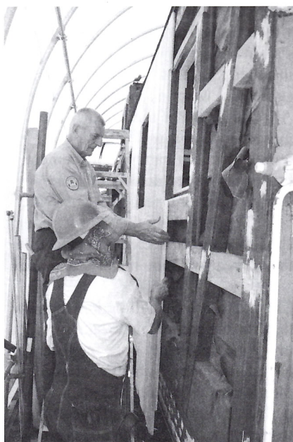
In Chama David Priddle (from the UK) and Mike Thode replacing siding on caboose 0503.
