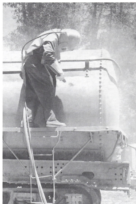
Chuck Armstrong sand blasting one of the tank cars on the RIP track in the east yards at Chama.
