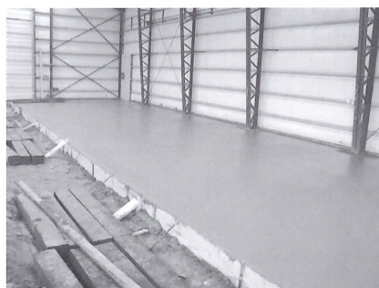
The finished floor of the CRF. Twenty-nine yards of concrete were poured. (Ted Smith)
