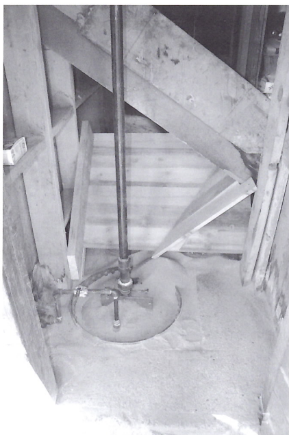
Inside the sand house in the Chama yard, the new sand chute built by the wood shop team is in place. (Tom Cardin)
