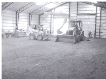
A contracted backhoe operator digs down the floor of the Antonito CRF to the level that ties and rail will be installed, which will be the bottom level of the concrete forms. (Ted Smith)
