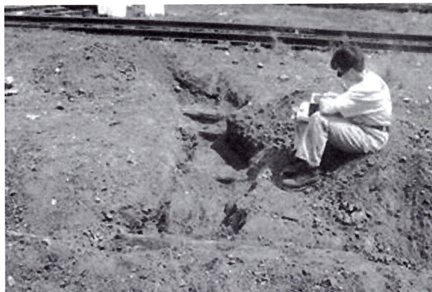
Team leader Laura Kammerer documenting evidence of coal bunker foundation members at the south end of the new snowshed. Flanking the snowshed, two such structures were constructed in 1916 on the site of the former covered turntable.
