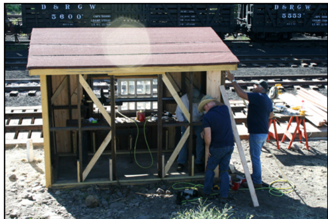
Tongue and groove siding is being installed on the west wall.
