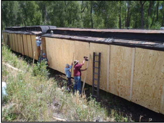
Putting 5/8" 4'X8' sheets of plywood on the siding of the 3 cars.
