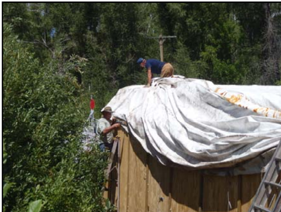
Putting temporary covering on the roof.
