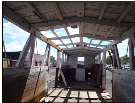
Rotted roofing has been removed.
