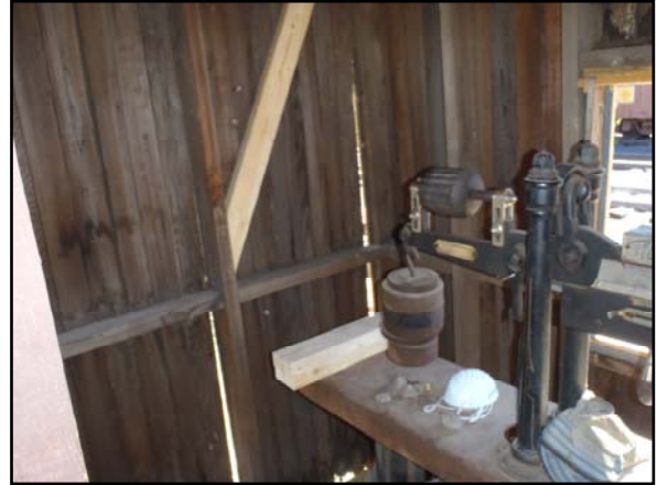
Cross bracing being installed on the interior walls
