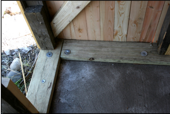
Floor sills have been replaced and secured with concrete nails
