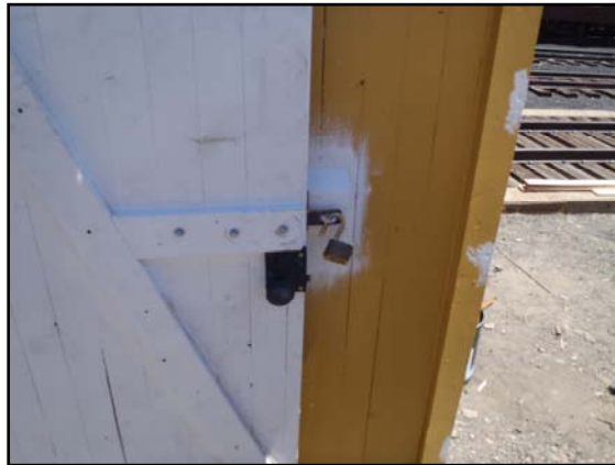
The hinge and hasp have been re-installed.
