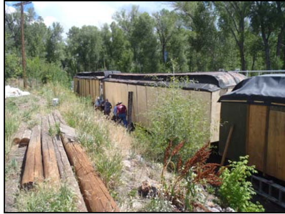
Putting 5/8" 4'X8' sheets of plywood on the siding of the 3 cars.
