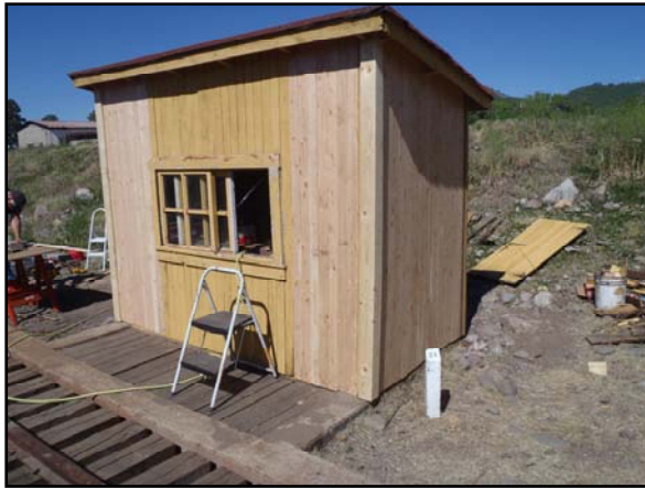
Shows new corners and old wood that was saved and reused.
