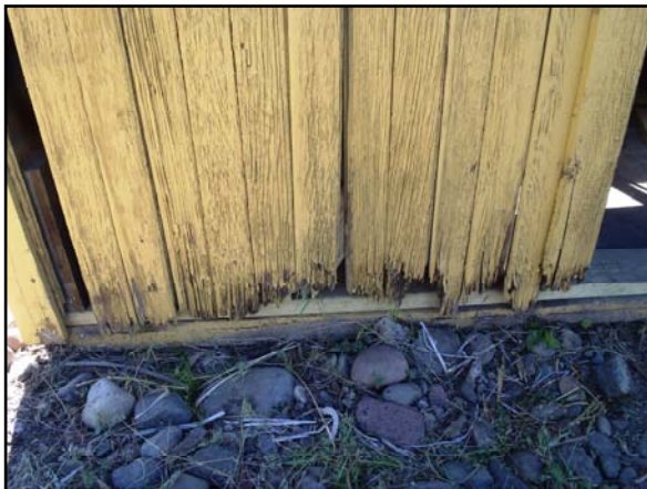
Old rotted siding before it was removed.
