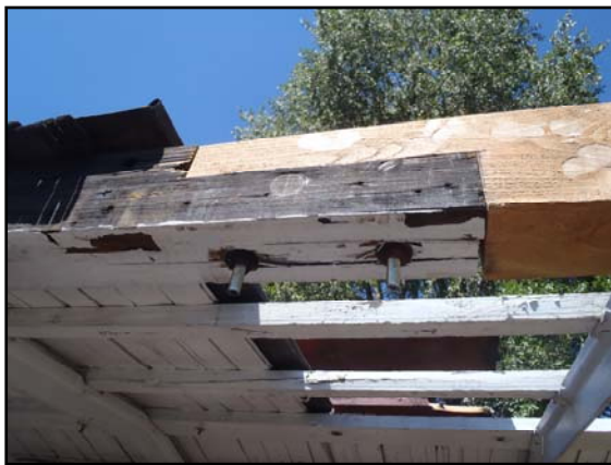
New header has been spliced in the middle of the car.
