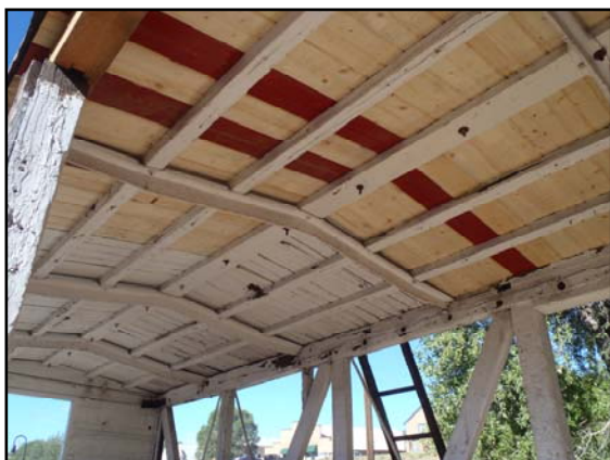
Roof boards have been replaced.
