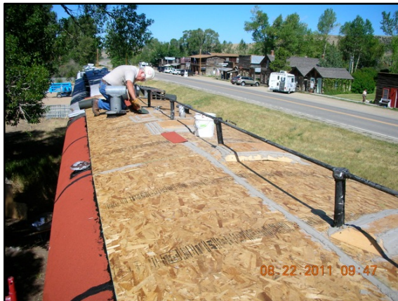
Chuck Deuker working on the A-3 Roof – note the raised penetrations covers.
