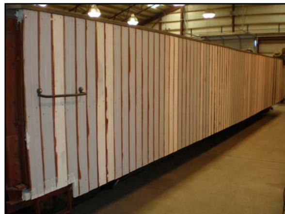
Siding installed. All tongues were painted prior to installation.
