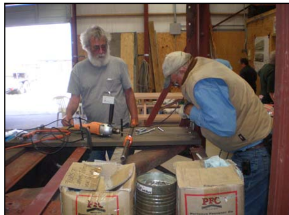
First two TREX boards being bolted down.
