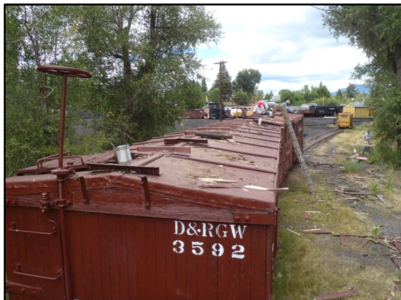
Roof walks being removed from #3592 and #3669.
