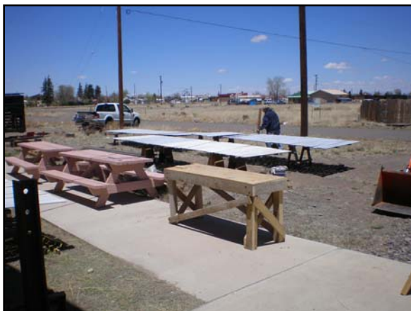
The siding was primed prior to installation.
