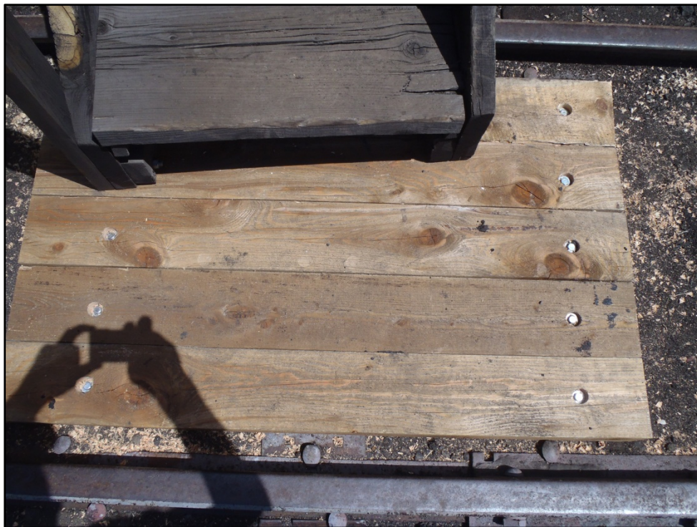
Wooden platform installed between the track for safety.
