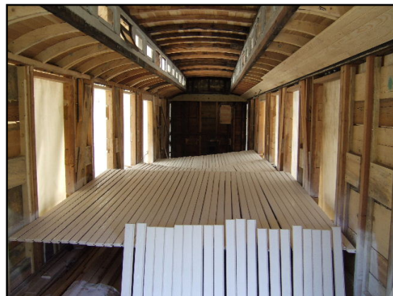
Painting with primer inside surface of exterior siding.
