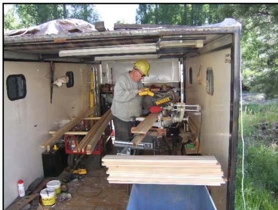
Don Storm cutting exterior siding.
