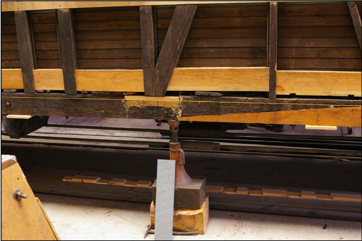
Area to be reinforced with steel on inside of sill.
