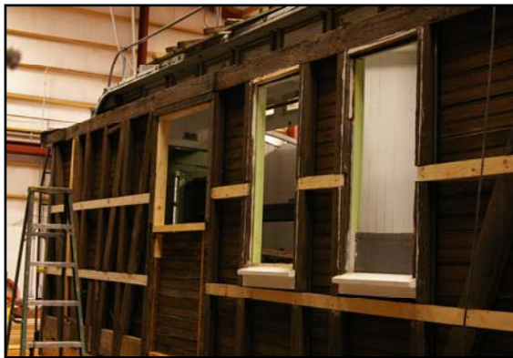
Old windows removed, note sill at differing heights.
