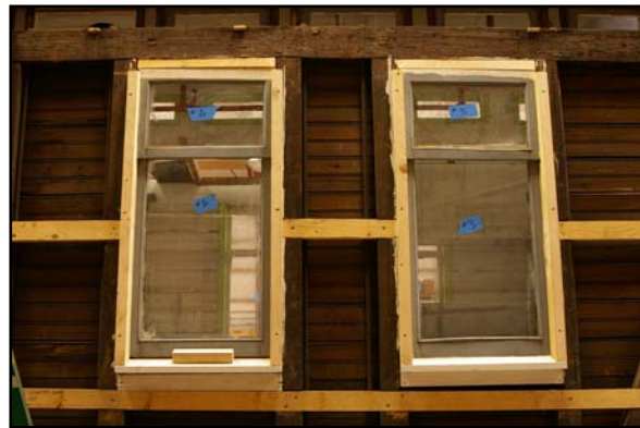
New windows installed with new deeper guides
