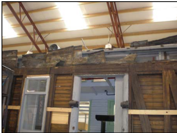
Roof tin in the process of being removed.
