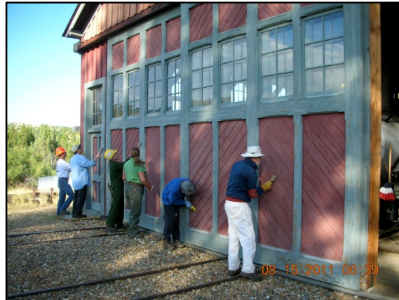
Painting prep work consisted of scrapping, wire brushing and pressure washing each building. Right to left, Roger Breeding, Noreen Breeding Karen Rahne, Mac Palmer, Tim Tennant and Bill James.
