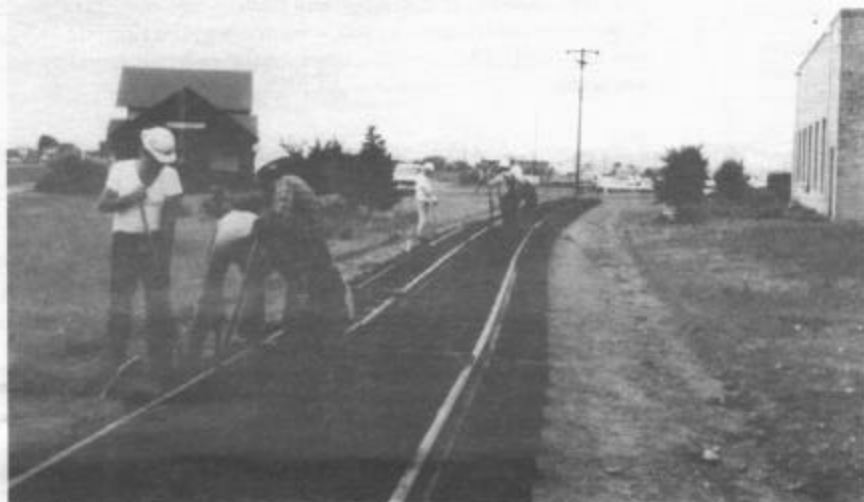
ABOVE: Laying track at Antonito. Four separate crews were working at once. One group joined the rails; another group spiked the first standard-gauge rail; the third group, shown in the foreground, gauged and spiked the other standard-gauge rail; and the fourth group, in the background, gauged and spiked the narrow-gauge rail.
