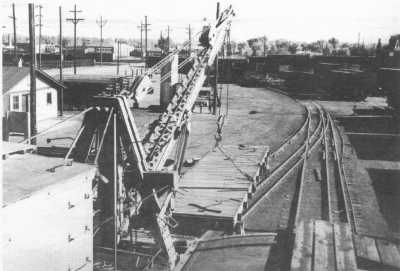
Derrick OP loading experimental flatcars for shipment to the U.S. Army, Alamosa, Colorado, 1955. Note that the boom tender flat 06063 is parked elsewhere when the derrick is operating. Photograph by Robert Richardson, Colorado Railroad Museum, used with permission.
