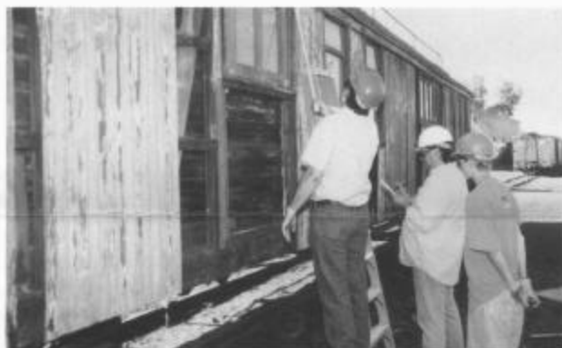
At the first session, from left, James Sutherland, Tony Kassin, and Craig Sutherland inspect cook car (former Railway Post Office car) 053 parked in Chama. Having done an inspection of the exterior in 1996, they needed to know more about the structural condition under the siding. The siding was removed at two-foot intervals, revealing a 112-year-old car in very good shape. Windows were removed to get a detailed picture of the frames that will need to be replaced, and plans were made to replace the eighteen screen frames in the clerestory roof. The roof was inspected and found to be in very good condition.
