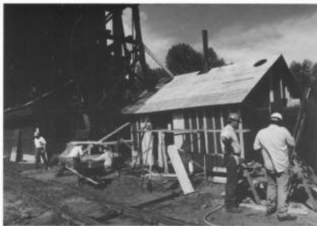
The sand house in the Chama yard with the new plywood roof sheeting, siding, and battens.
