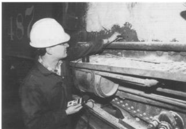
Walt Rosenberger uses an ultrasonic device to measure boiler thickness on the 487, January 1999. Tom Atkinson (not shown) is also a member of the Chama enginehouse crew.
