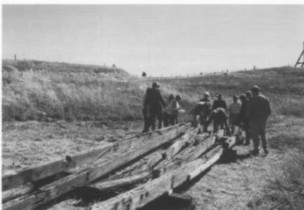
Rotten longitudinal sills from flat car 06008 outside the Friends' facility at the Western Museum of Mining and Industry in Colorado Springs, October 1998. Art Nichols photo.
