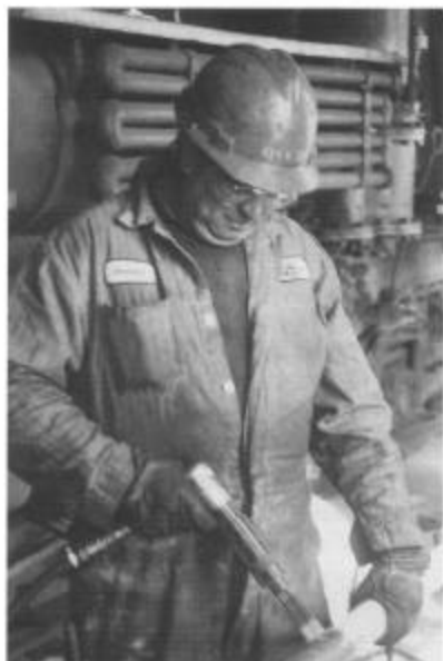
Donald Martinez uses a needle gun to descale flue tubes, January 1999.
