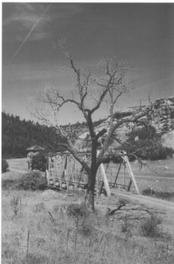
Through-truss bridge and water tank at Navajo, MP 377.7, thirty miles west of Chama. The bridge, which crosses the Navajo River, is the same design as the Chama River Bridge on the C&TS. There was also a 23-car siding located next to the water tank. August 1993, Art Nichols photo.
