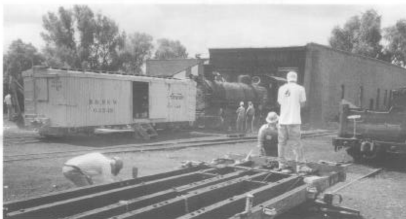
New end sill being installed on rail and tie car 06051. Parked in front of the old roundhouse are newly lettered outfit car 04549 and, awaiting major boiler work, engine 488 with lagging removed (session B). (Photo by George Swain.) Below, restoration continues on the Osier section house (session A). (Photo by Tom Cardin.)
