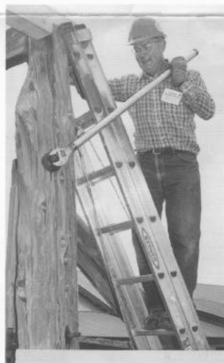
George Berkstresser uses a “cheater bar” to loosen the nut holding the hinge for one of the gates on the stock pens at the Chama wye (session A).
