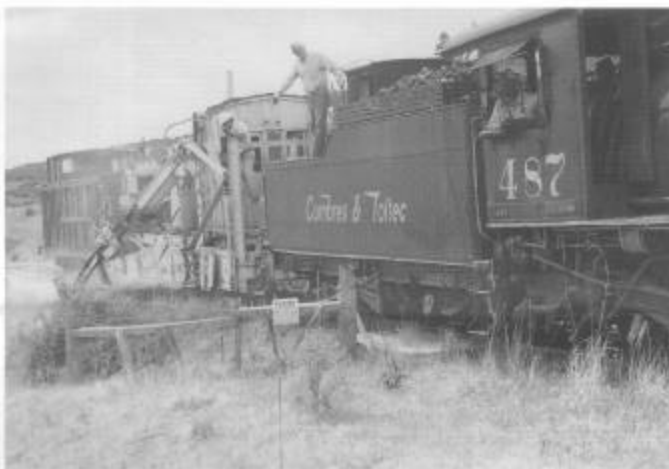
The Jordan spreader taking out weeds along the track, just east of the Highway 17 crossing below Coxo. (Photo by Tom Cardin.)
