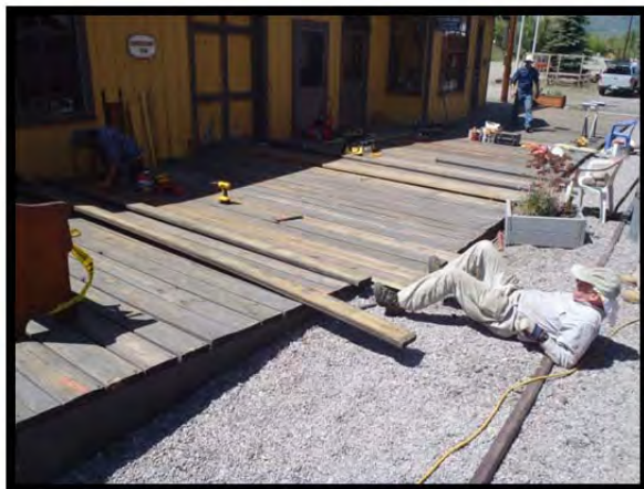
Ron Lira screws down new plank as Dr. Alan Robson holds the plank tight with his foot.
