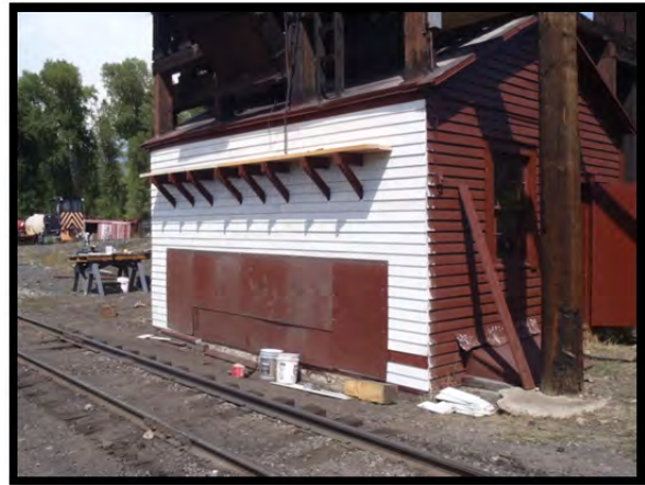
West side residing completed except for except for painting.
