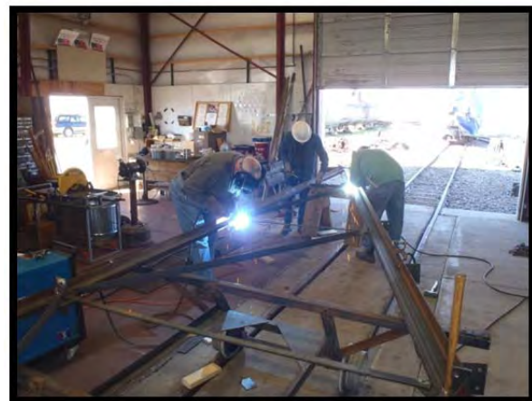
Marshall Smith and TL Russ Hanscom welding angle iron cross bracing while Rod Whelan hold a piece in place.
