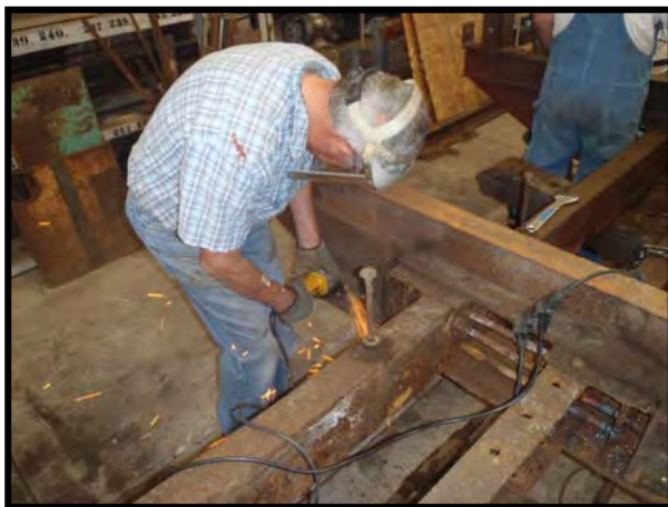
TL Bill Pratt grinding off a rivet head.
