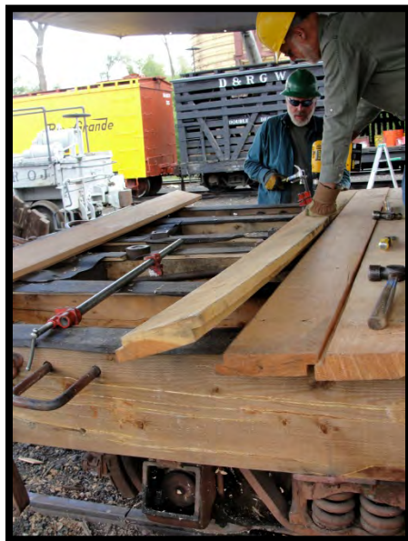
Badly warped lumber is hard to work with. 97
