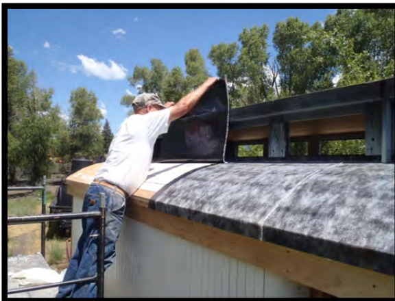
TL Don Bayer putting down Ice and Water shield – a rubberized fiberglass material.
