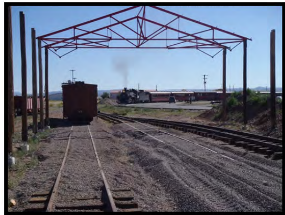
First pair of trusses bolted into place as the afternoon train arrives from Chama.
