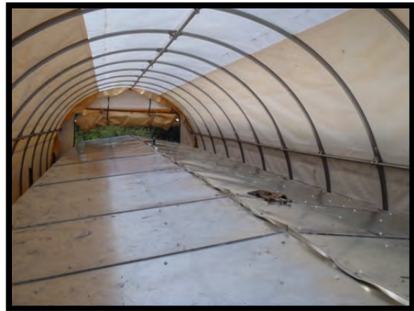
Finished metal roof – the roof walk was also added.
