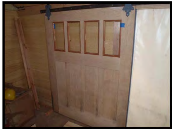
A new entry door temporarily hung to be removed at a later date for painting.
