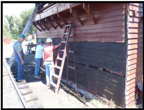
Sam Schechter, Rob Reib and Ron Schmitt removing west siding.
