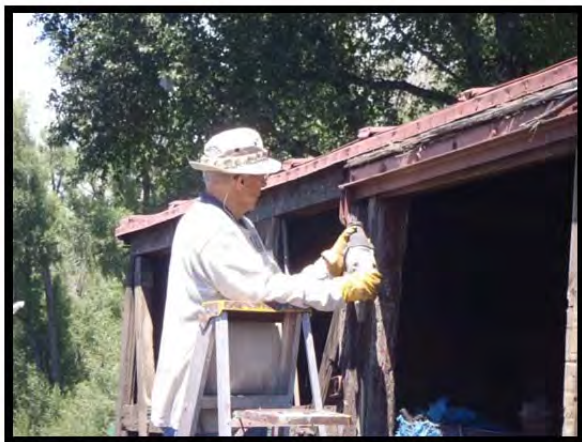
George Davies uses a “sawsall” to cut a bolt.
