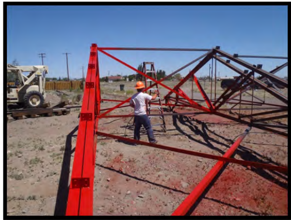
Chase Kepner spray paints an assembled pair of trusses.
