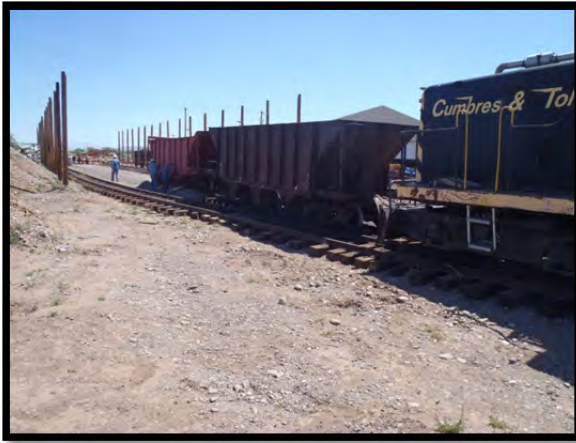
The railroad has just finished dumping ballast on the center track.
