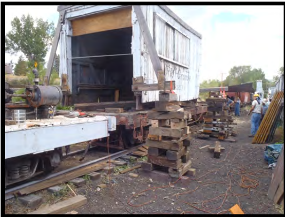
OP's cabin has been raised by cribbing to clear the flat car so it can be moved out.
