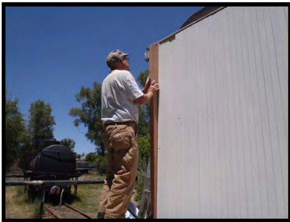
TL Don Bayer checking the fit of a corner post.
