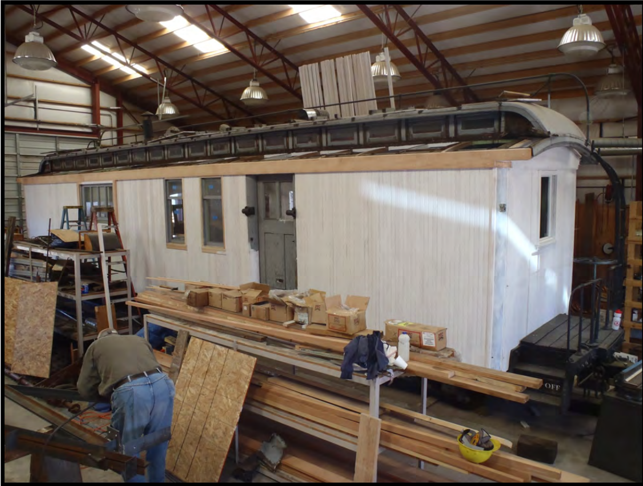
Car at the end of Session B. Both sides and both ends were completely sided during Sessions A & B.
