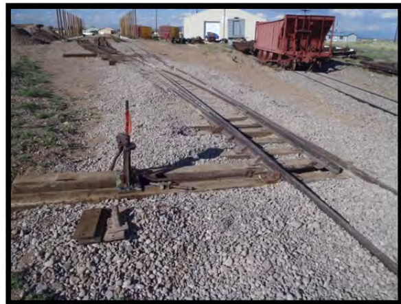
Switch Stand and throw rods installed.
