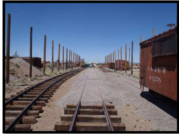
Without the ballast the fork lift would not have been able to straddle the track & ties.
