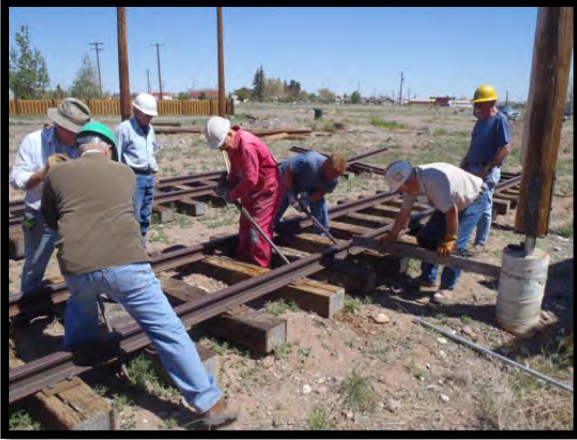
Team aligning track. It doesn't take much of this type of work to wear you out!
