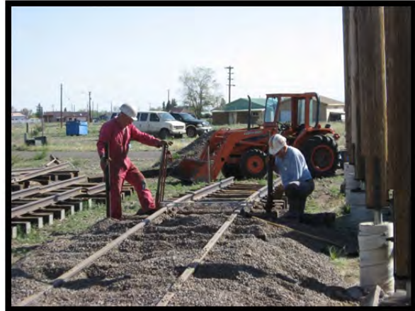
Raising the track to grade using a couple of "Handy Man" jacks.
