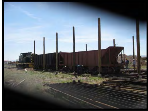
Railroad unloading ballast on Track 1.
