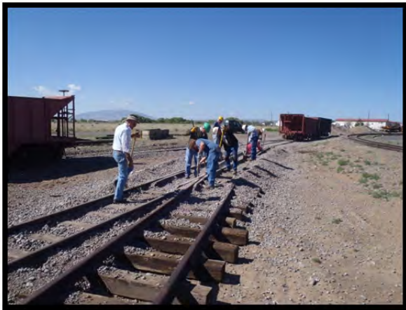
Team removing ballast so switch stand and throw rods could be installed.
