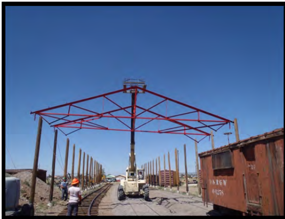
First pair of trusses being moved into place.
