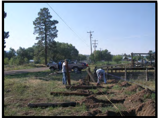
Digging holes for the posts. (Photo by Len Jones)
