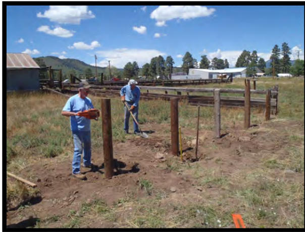
TL Len Jones cutting post to right height. Jim Sublett fills in around a post.
